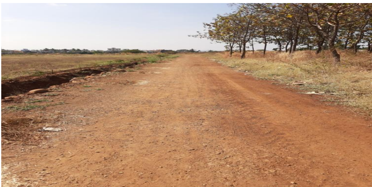
Road built up by use of construction waste
