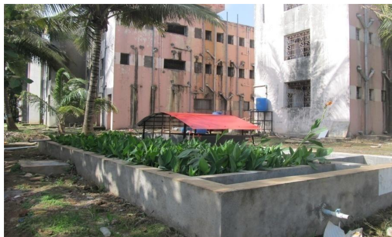
Wastewater treatment in the phytoremediation tank
